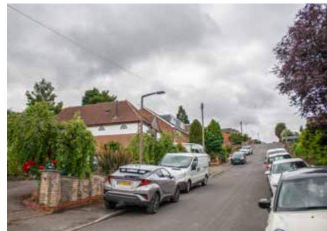
Residential development on a steep slope at Standhill Avenue
